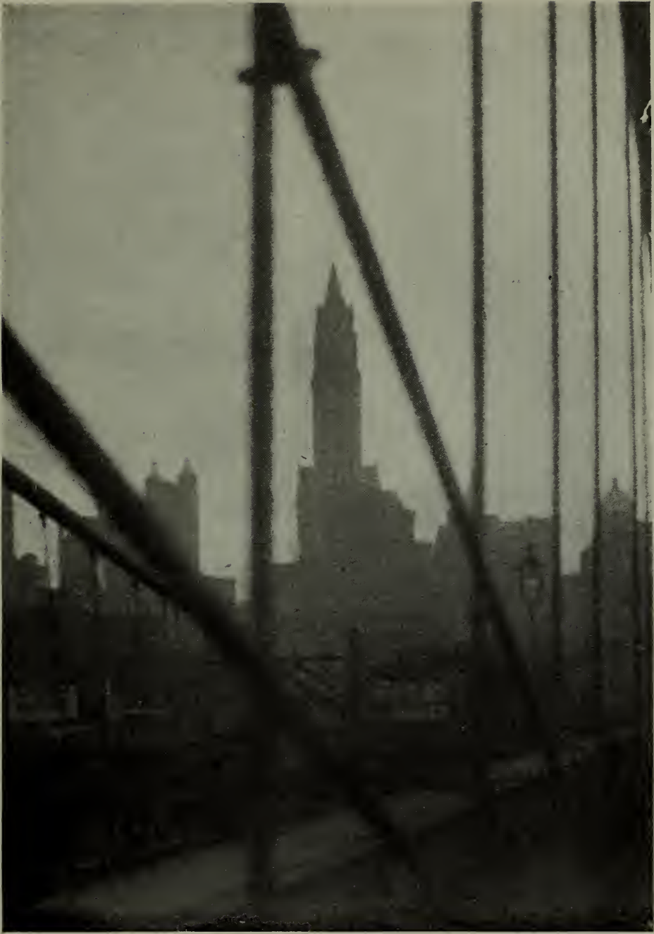
THROUGH THE CABLES OF BROOKLYN BRIDGE.
